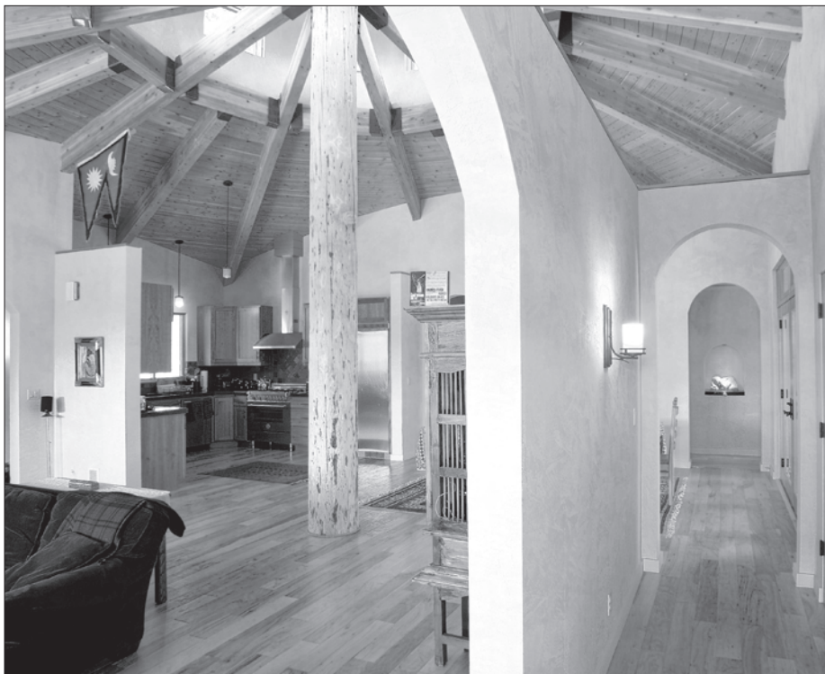
A Douglas fir trunk braces beams that support the circular roof. The clerestory windows above, which open with the push of a button, allow for natural ventilation.
